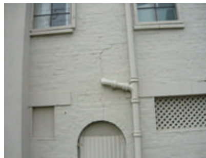
Door to public male toilet note cracking of brickwork down face of wall at angled downpipe
