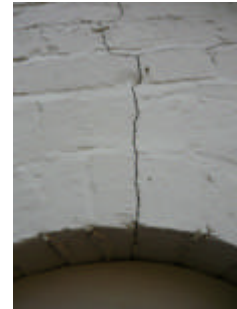
Crack in brick arch above toilet door
